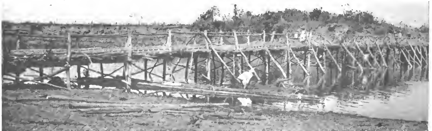
Cart bridge formerly at Cabanatuan over which thousands of carts of rice were hauled in harvest time. This type of bridge is strong enough to carry a loaded 3000-lb. touring car. Most of these structures have been supplanted by collapsible deck bridges, the flooring of which is attached to one bank by heavy cables so that when the river rises this floor or deck is lifted off the piles and swung to the shore. When the water subsides replacement is easy
